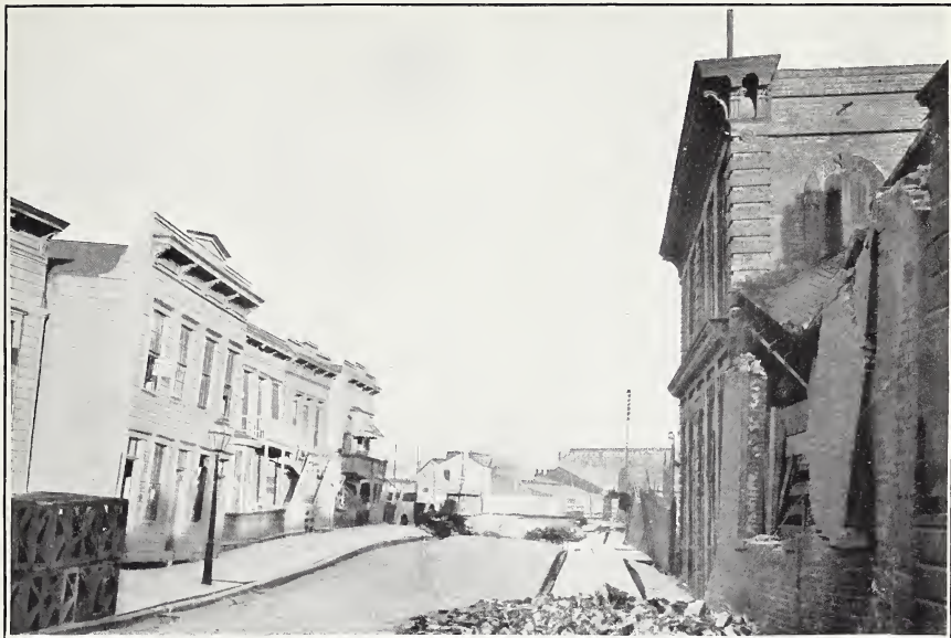
A. SETTLING (5 FEET) ON DORE STREET, BETWEEN BRYANT AND BRANNAN STREETS, SAN FRANCISCO.
